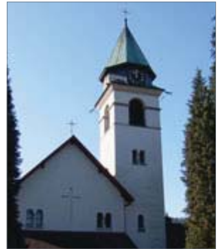
Church with AFILS system installed
